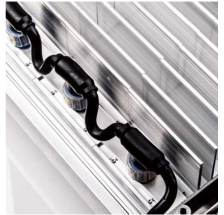
New module connection, neat, clean more efficiency
